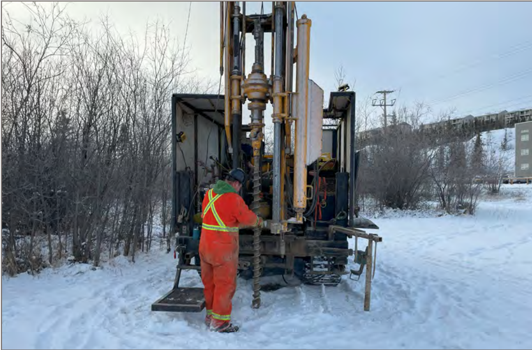
Photo 3: BH24-01 - drill setup, facing southwest.
