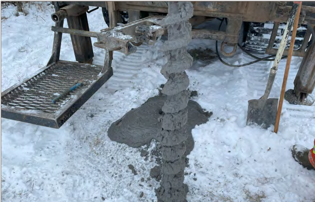
Photo 4: BH24-01 - Auger run (1.5 to 3.0 m depth).
