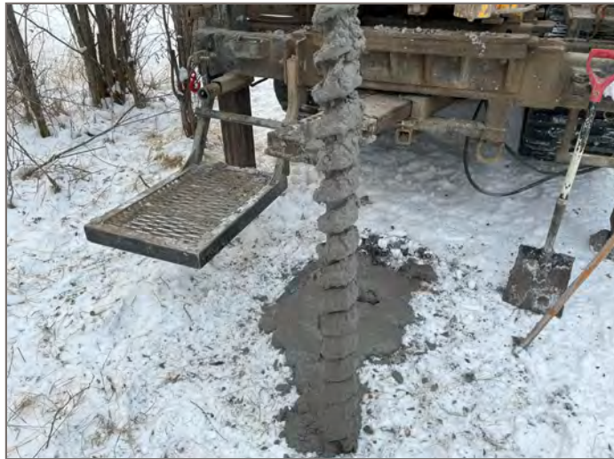
Photo 5: BH24-02 - Auger run from 1.5 to 3.0 m in depth; Sand, silty, fine grained, greyish brown.
